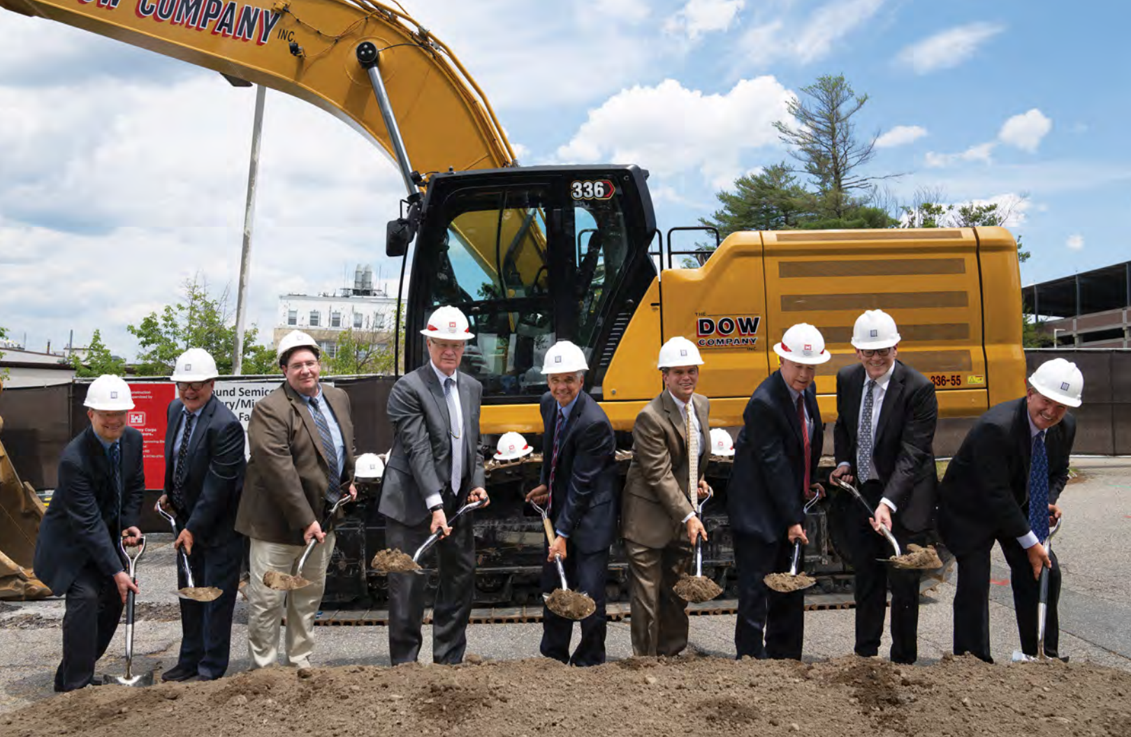
Members of the CSL-MIF planning team—(left to right) Kriss Pettersen, David Pronchick, Mike Menadue, Alan Shaffer, Eric Evans, Scott Anderson, Bob Baker, Israel Soibelman, and Craig Keast—break ground for the new facility on July 11.
