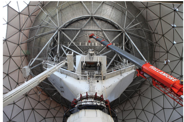
FIGURE 6. A crane connected to the 30-ton counterweight compensates for the missing RF box as the antenna is rotated to zenith for the last time.
