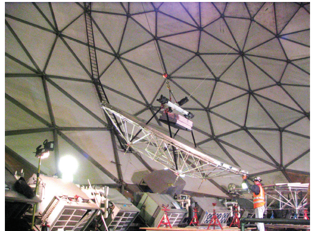
FIGURE 43. A subframe is lifted off the control room roof.
