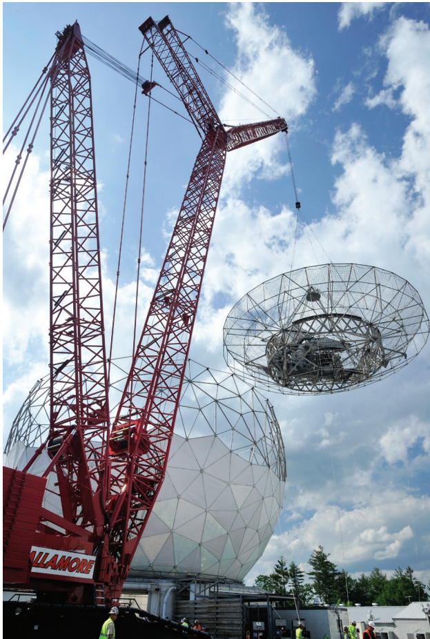
FIGURE 15. The 43-ton old backstructure was lifted over the edge of the radome and set down behind the temporary building to await demolition.
