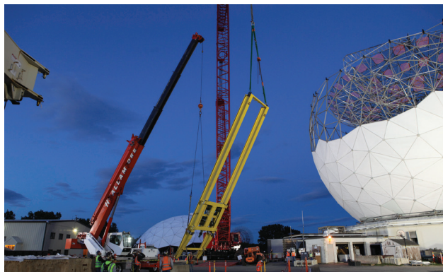
FIGURE 33. The rails and dolly for the RF box insertion system are raised up in preparation to be threaded down into the transition structure.
