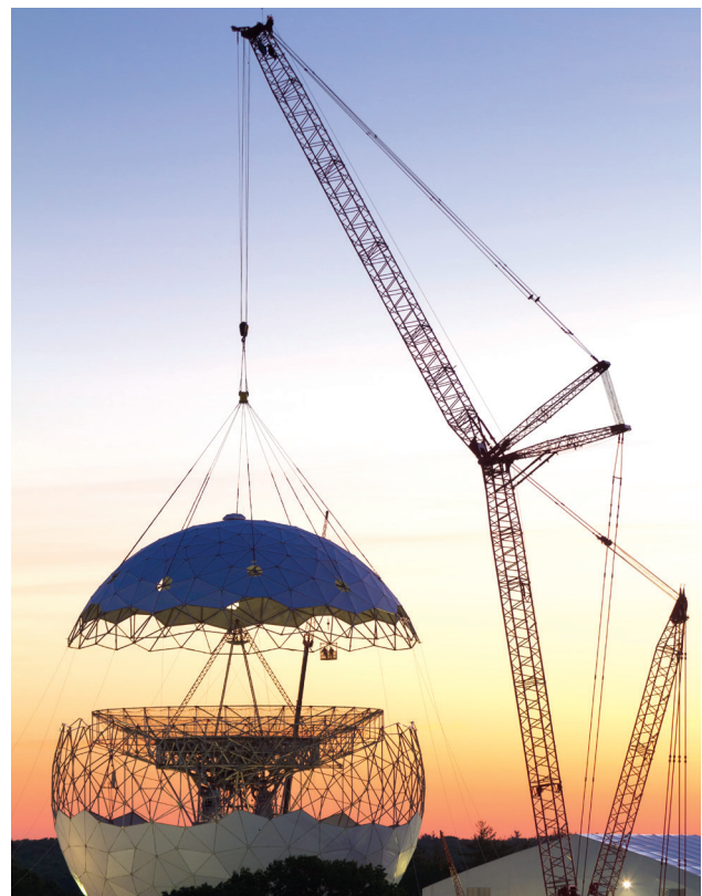
FIGURE 13. The 400-foot-tall main crane and smaller support cranes are silhouetted against the sunrise just after the radome cap is lifted. Photograph by Colin Lonsdale.
