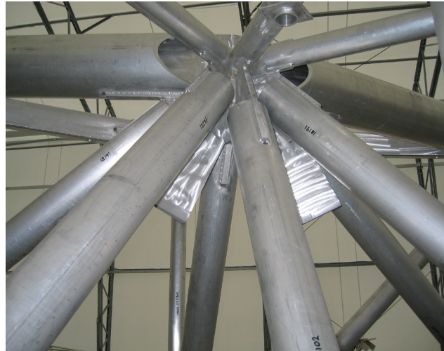
FIGURE 27. This node point has 13 connecting elements.
