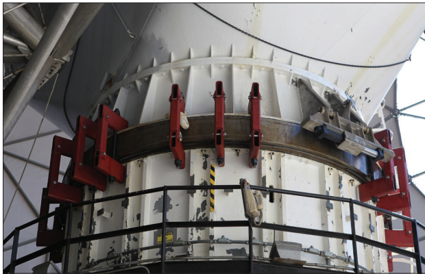
FIGURE 8. The 200 lb clamps around the azimuth bearing ensure that the antenna does not tip over when exposed to high winds.
