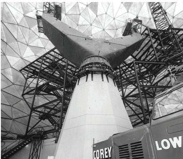
FIGURE 2. Mobile cranes and extensive scaffolding were used to build the original Haystack antenna within the confines of the radome.
