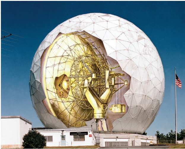
FIGURE 4. This rendering is a cutaway view of the old Haystack antenna that shows the RF box being lowered.
