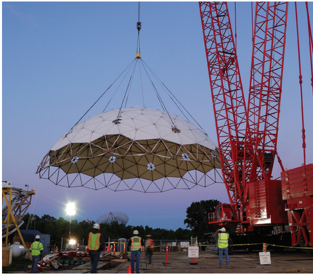
FIGURE 14. The cap was lifted off the Haystack radome and carefully swung to its temporary landing site.
