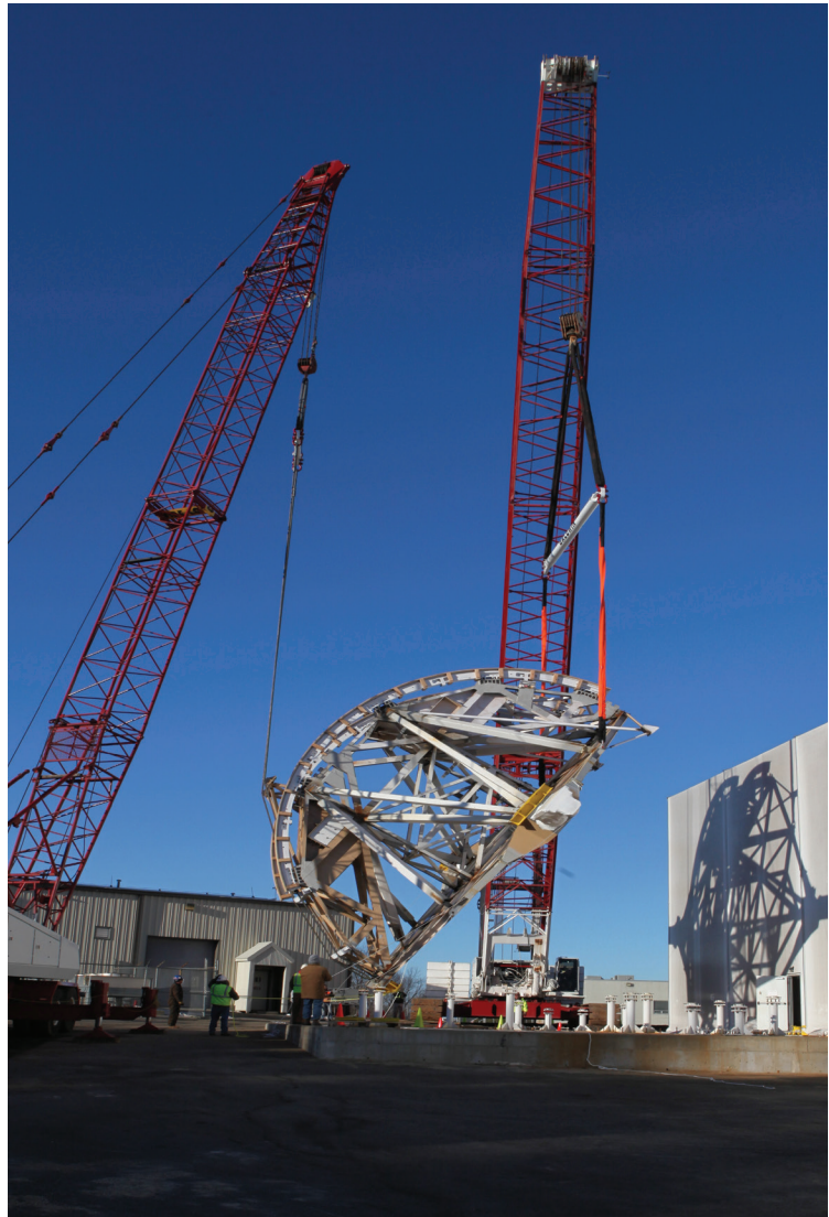
FIGURE 23. During a tandem lift operation, the transition structure is inverted and moved from its face-down assembly area to a pair of supporting tripods where final integration continues face up.
