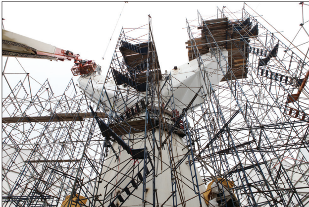
FIGURE 19. Towers of scaffolding ascend from the floor of the radome as the yoke structure is stripped of old components and modified to accept the new transition structure.
