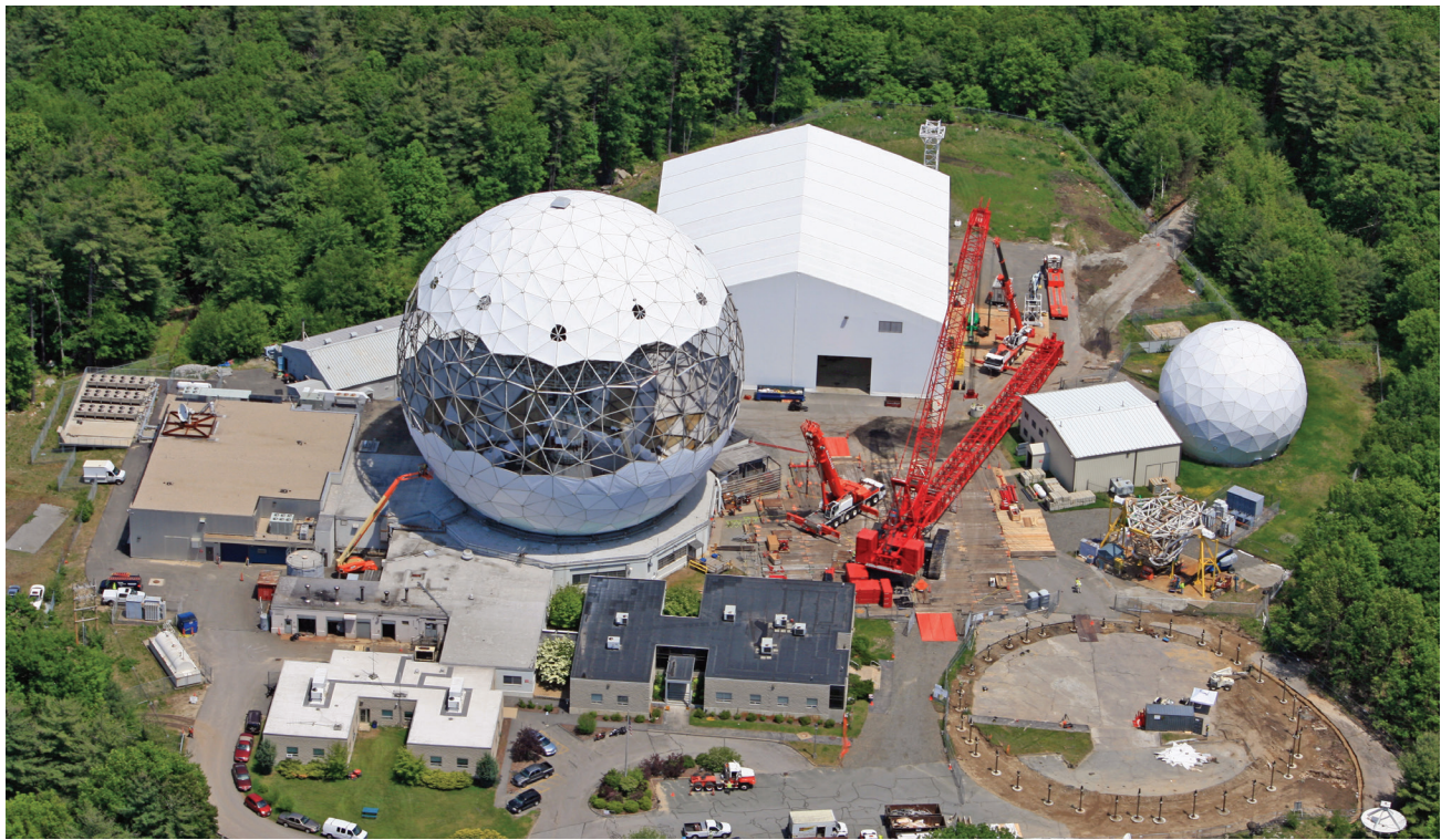
FIGURE 11. The assembly of the heavy-lift crane takes place along a 400 ft roadbed built into the treeline while the radome membranes around the equator are removed in preparation for the separation of the radome cap. The temporary landing zone for the cap is the ring of steel piers in the lower right corner.
