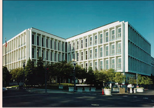
FIGURE A. The Hart Senate Office Building was the scene of the Ba attack on October 9, 2001.
