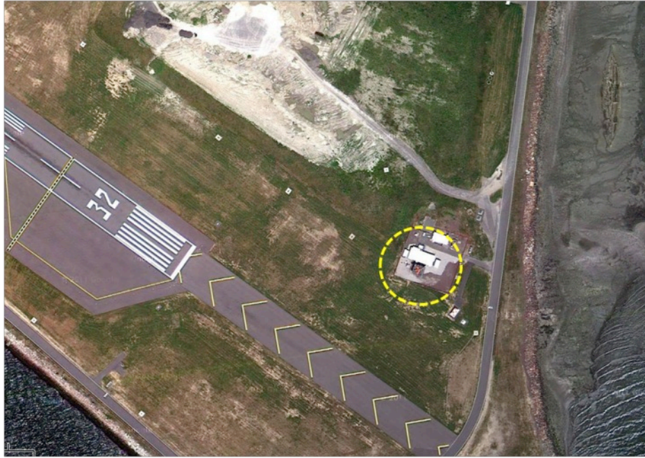
Figure 4-4. ASR-9 site at Logan International Airport in Boston, Massachusetts.
