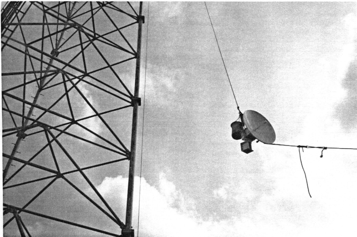
Figure 5. MTS being hoisted to the 170-foot-high tower.
