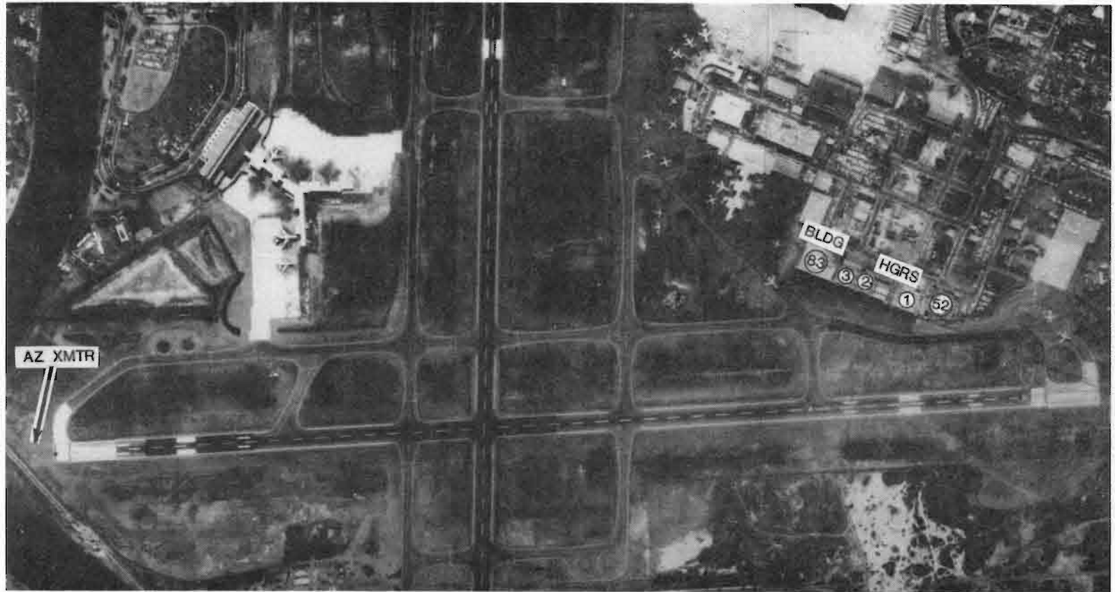
Fig. 3-96. Aerial photograph of Sydney Australia runway 07-25.
