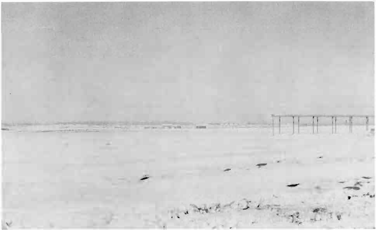
Fig. 4-4. ILS localizer and McDonnell-Douglas buildings from St. Louis multipath measurement site.
