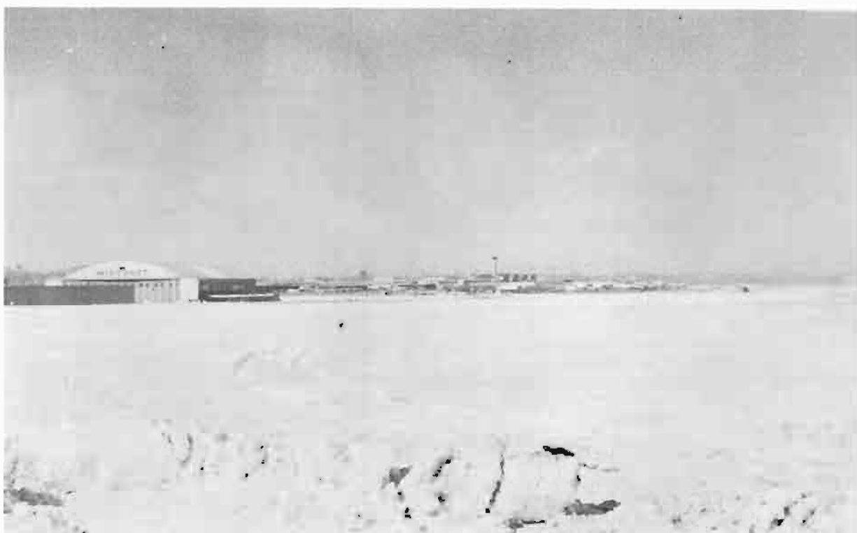
Fig. 4-5. St. Louis (Lambert) terminal area buildings as seen from measurement site.
