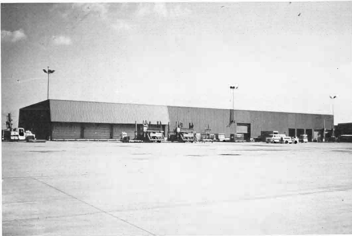
Fig. 7-3. United Airlines cargo building at PHL.
