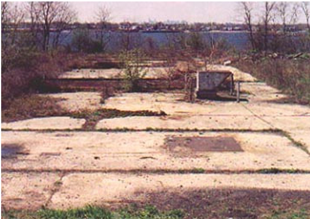
Figure D-3. The current picture of a former Nike missile launching facility at Hart Island. The foundation was proposed to be used as the TDWR foundation in initial site-survey documents. The Manhattan skyline is faintly visible in the background of the photo.
