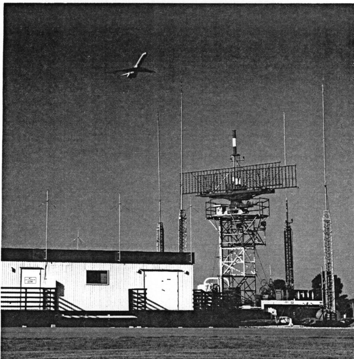
Figure 3-1. MIT Lincoln Laboratory PRM site at the Memphis International Airport.
