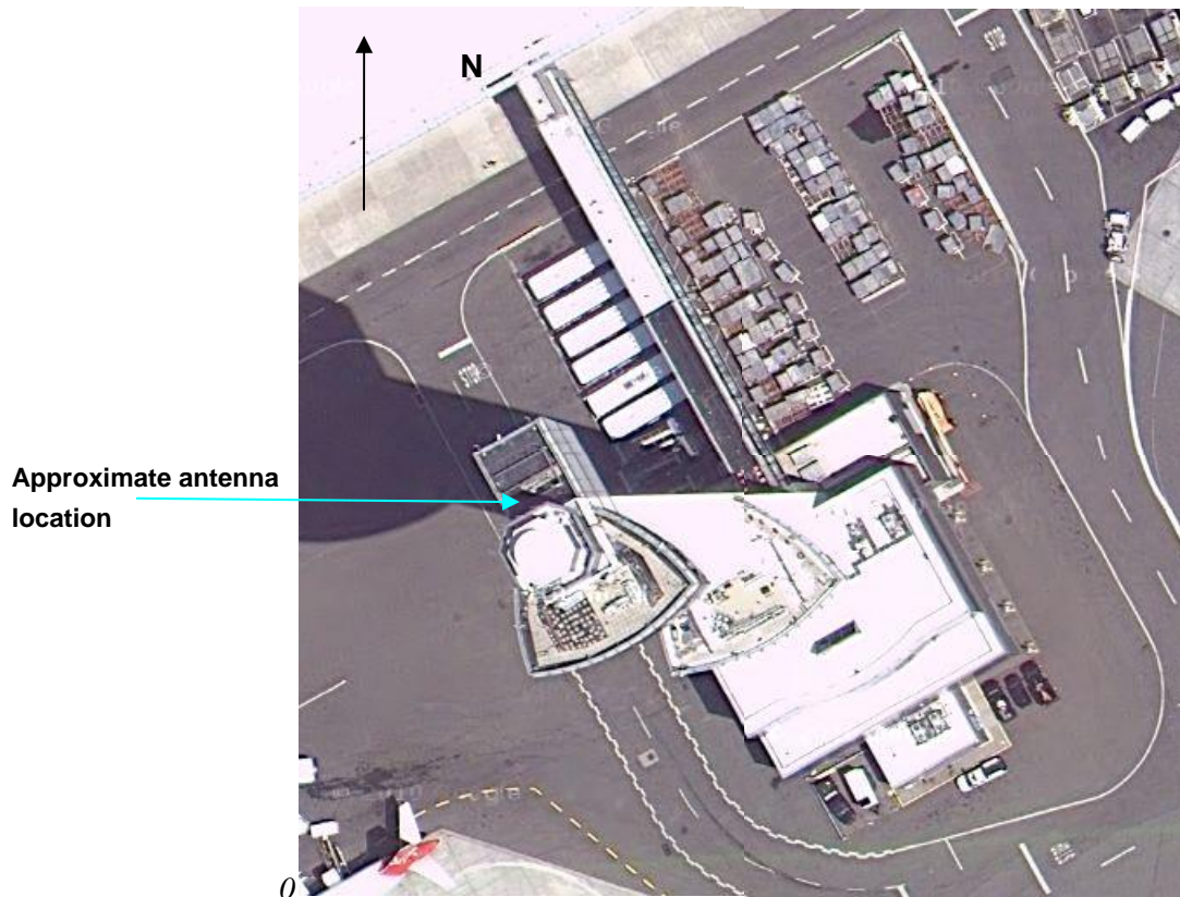
Figure 4. Another view of the tower and antenna location.
