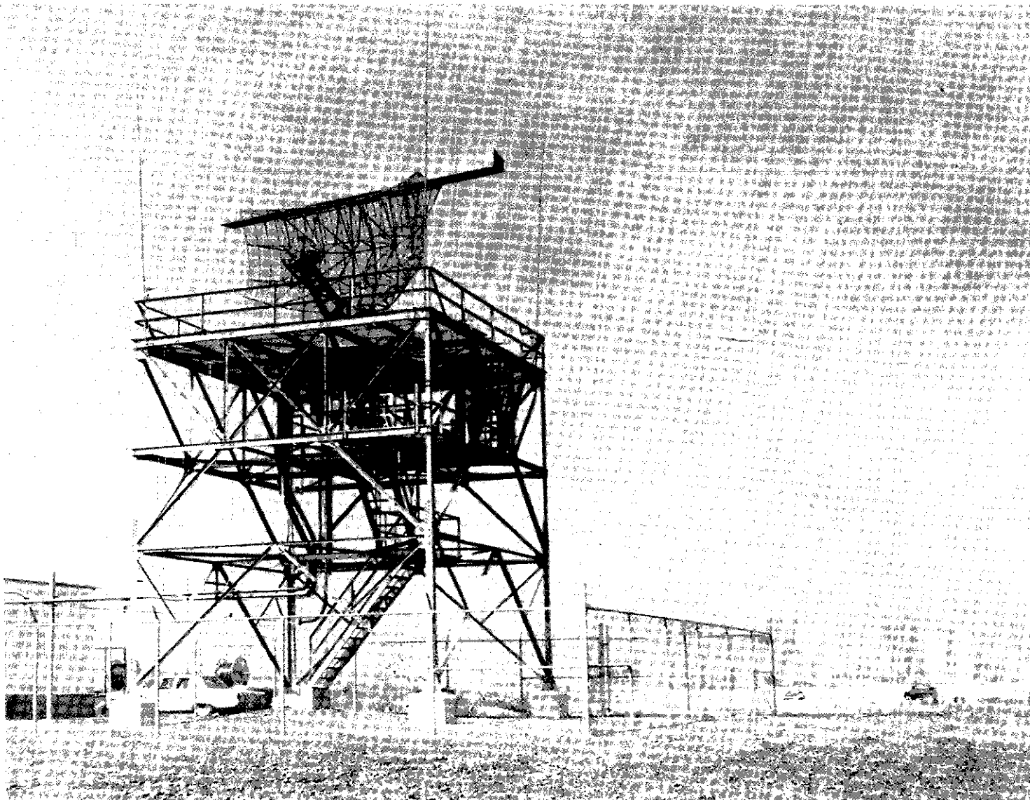
Fig. 14. ATCRBS hogtrough installed on ASR reflector.
