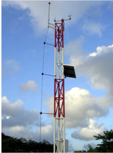
Figure 5-1. LLWAS tower with anemometer.
