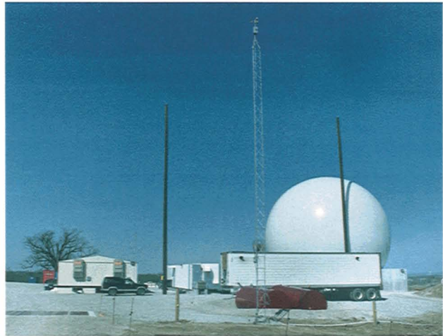
FIGURE 3. TDWR testbed located southwest of Kansas City International Airport.
