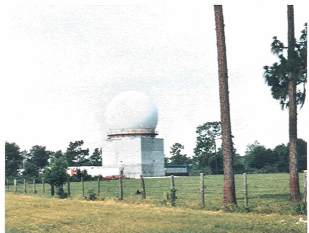
FIGURE 4. TDWR testbed located five miles south of Orlando International Airport.
