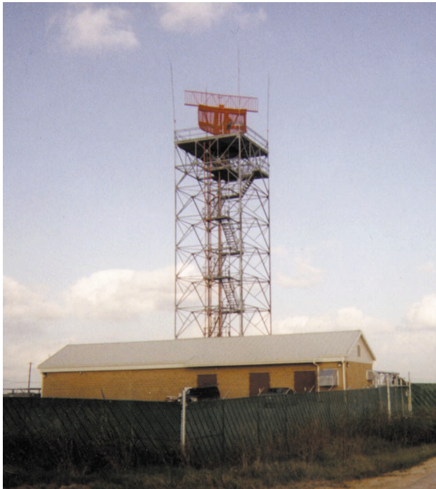
FIGURE 6. ASR-9 (above) at Austin International Airport in Texas, and components of the Lincoln Laboratory Weather Systems Processor (WSP) prototype (right). The WSP extracts microwave and timing signals from the ASR-9. A direct-down-conversion receiver and VME-based data processor provided fully automated detection of wind shear and storm tracking. Products are displayed to controllers in the tower cab and at the radar-approach control room.
